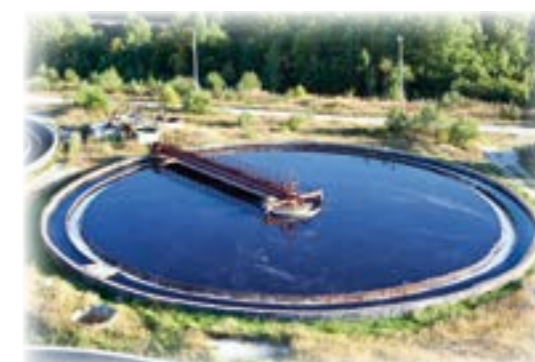
WASTE WATER TREATMENT
